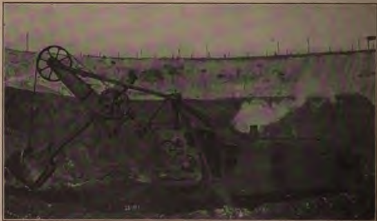
Atlantic Steam Shovel Stripping Iron Mine.
